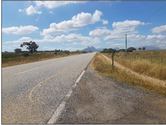
Pic 1 - Looking right (towards N1) from access (sight distance good)
