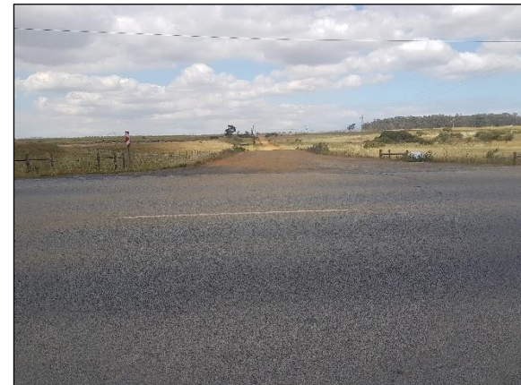
Pic 4 - Looking at farm access on R304
