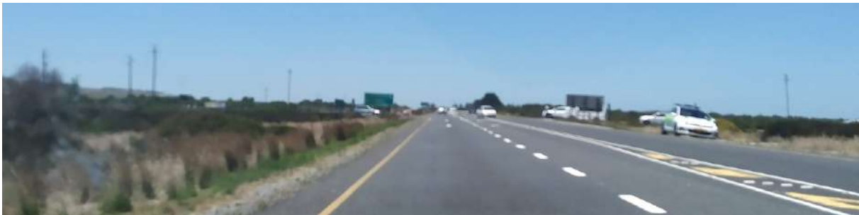
Photograph 4-17: View series southbound on the R27 approaching the R315 intersection.
