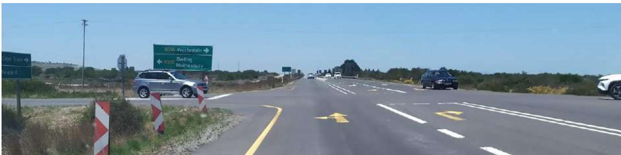
Photograph 4-18: View series southbound on the R27 approaching the R315 intersection.
