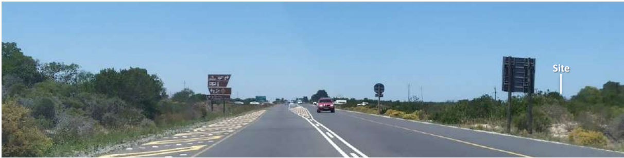
Photograph 4-15: View series southbound on the R27 approaching the R315 intersection.
