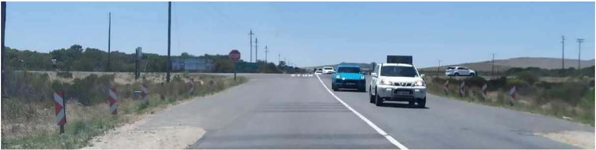
Photograph 4-24: View series eastbound on the R315 approaching the R27 intersection.
