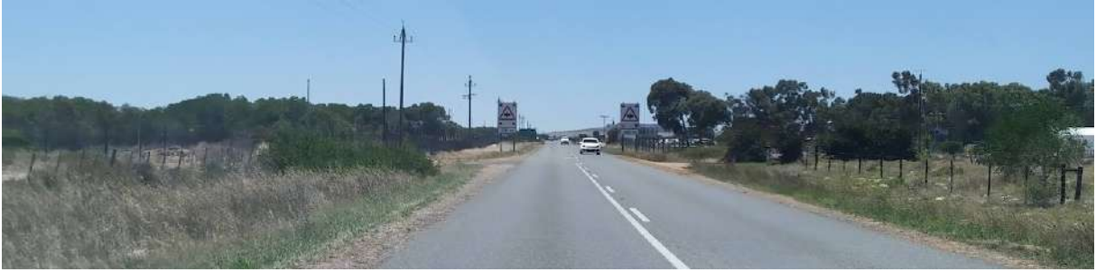
Photograph 4-23: View series eastbound on the R315 approaching the R27 intersection.
