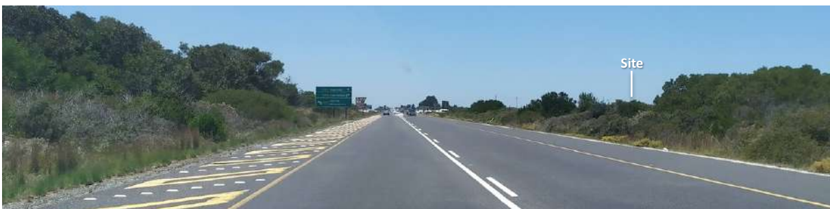
Photograph 4-13: View series southbound on the R27 approaching the R315 intersection.
