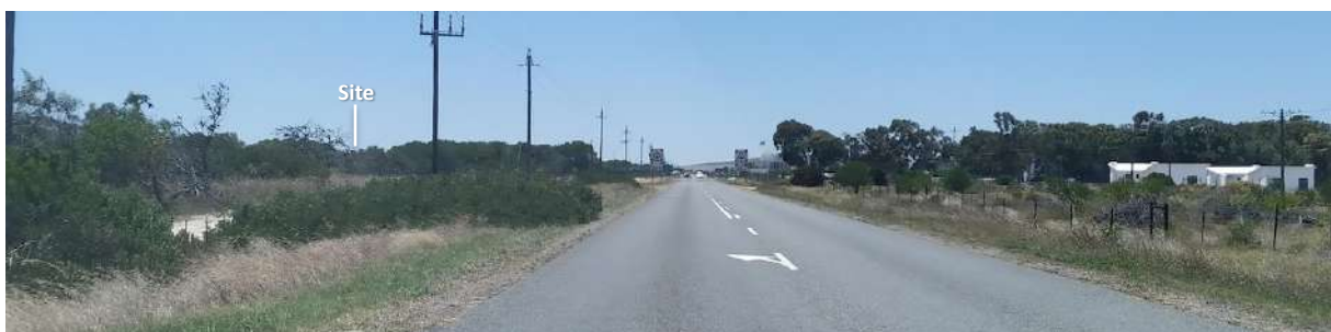
Photograph 4-22: View series eastbound on the R315 approaching the R27 intersection.
