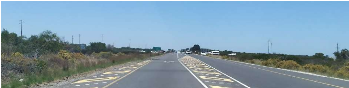
Photograph 4-16: View series southbound on the R27 approaching the R315 intersection.
