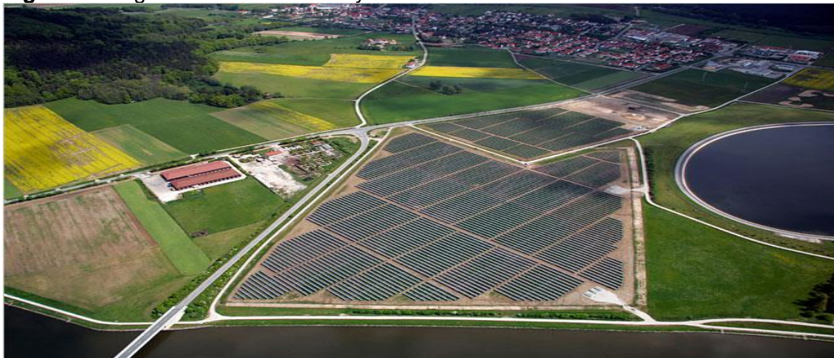
Figure 3. Aerial view of large scale Solar PV array
