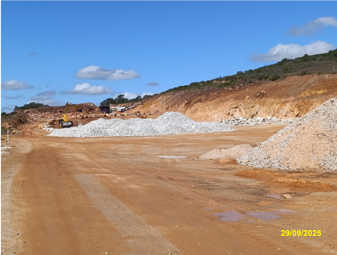
Photo 1: Existing 5ha mining permit area at foothill of Hoogmoed se Berg.
