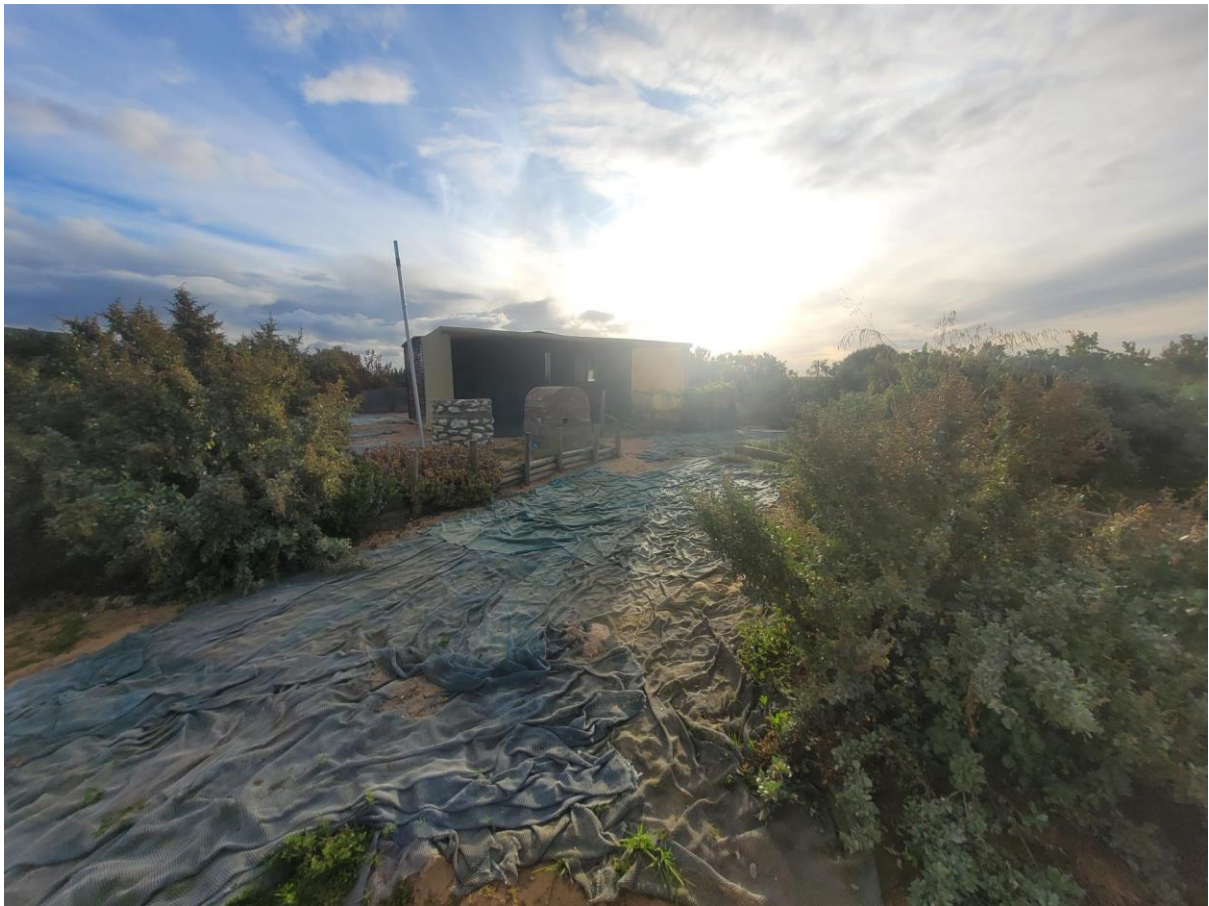
Photo 12: New Knor Varkie camp/caravan sites and facilities along existing road. (Photo taken 21/09/2023)
