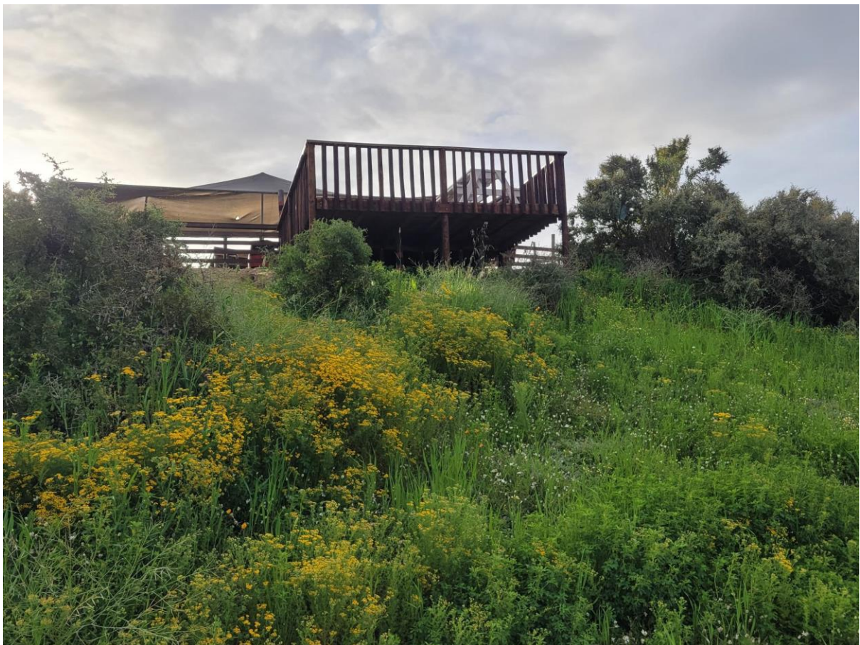
Photo 4: New deck as part of Knor Varkie Main Complex. (Photo taken 02/09/2023).
