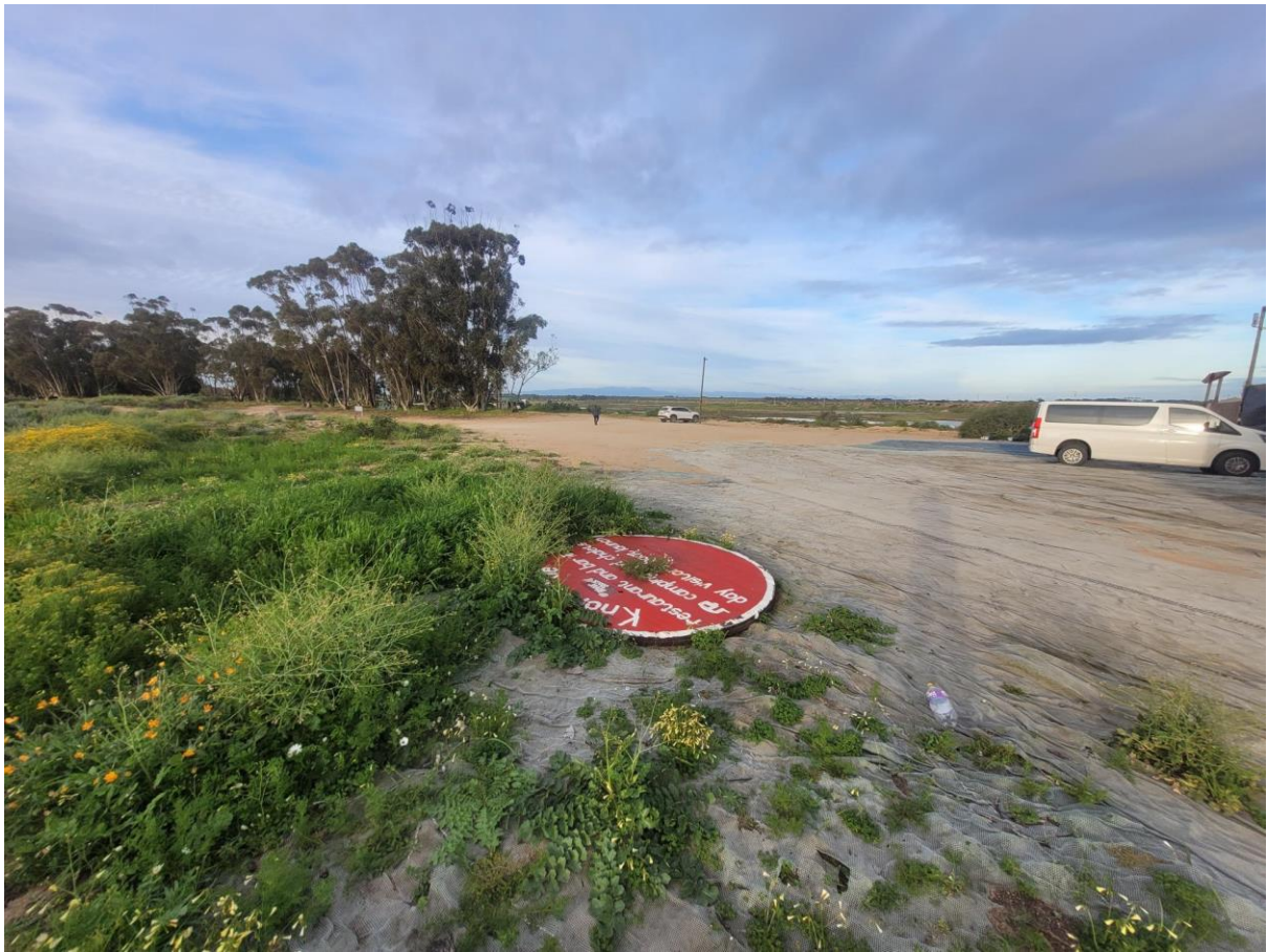
Photo 7: New parking area at new Knor Varkie Main Complex. (Photo taken 02/09/2023)
