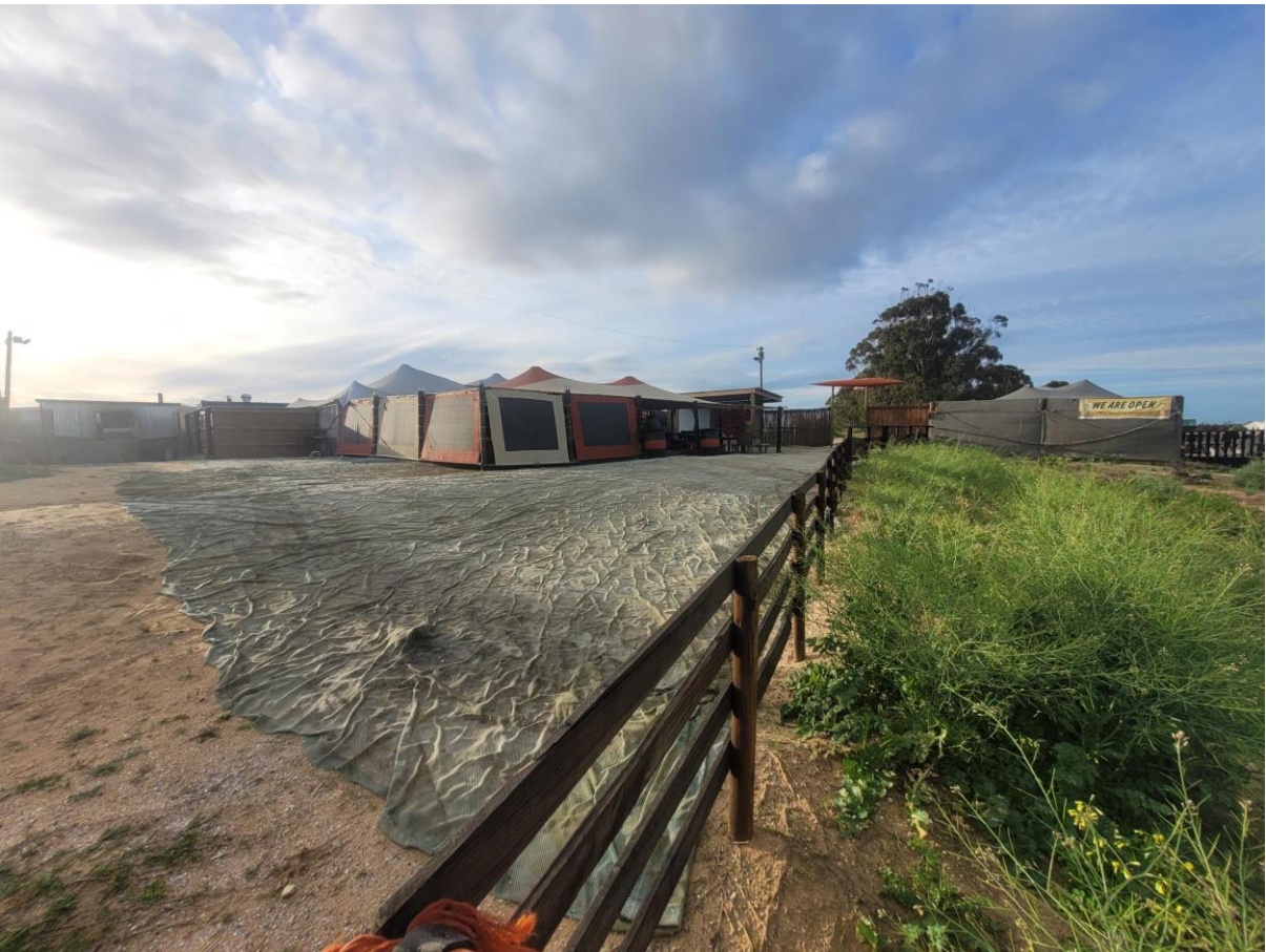
Photo 6: New Knor Varkie Main Complex. (Photo taken 02/09/2023).
