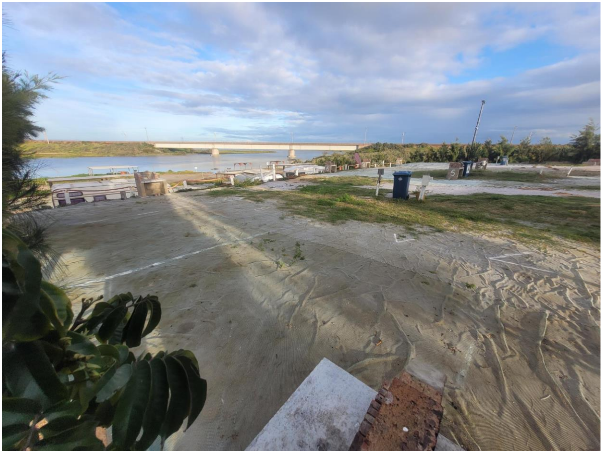
Photo 13: New Knor Varkie camp/caravan sites and facilities along existing road. (Photo taken 21/09/2023)
