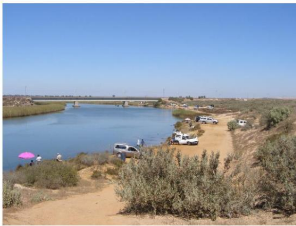
21) Control over area
