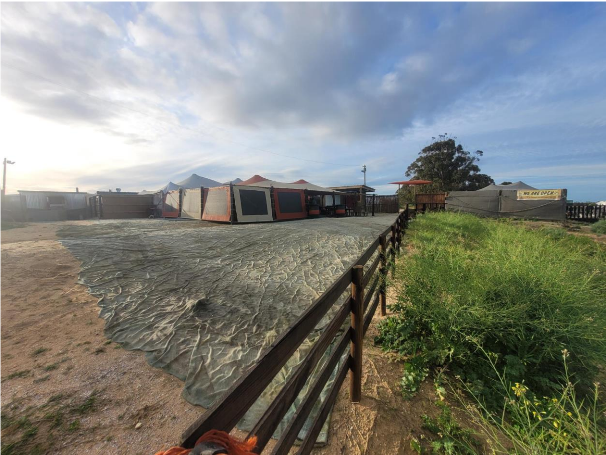
Photo 6: New Knor Varkie Main Complex. (Photo taken 02/09/2023).
