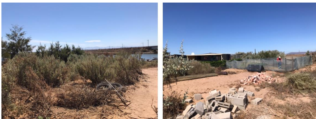
Figure 5.2. Building Rubble observed during site visit to Knor Varkie Resort. Left: wire. Right: Concrete and brick rubble.
