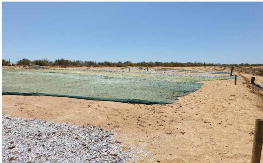
Photo 3: Camping area. Indigenous vegetation cleared. Mussel shells dumped. Area terraced to create different levels/areas for campers.
