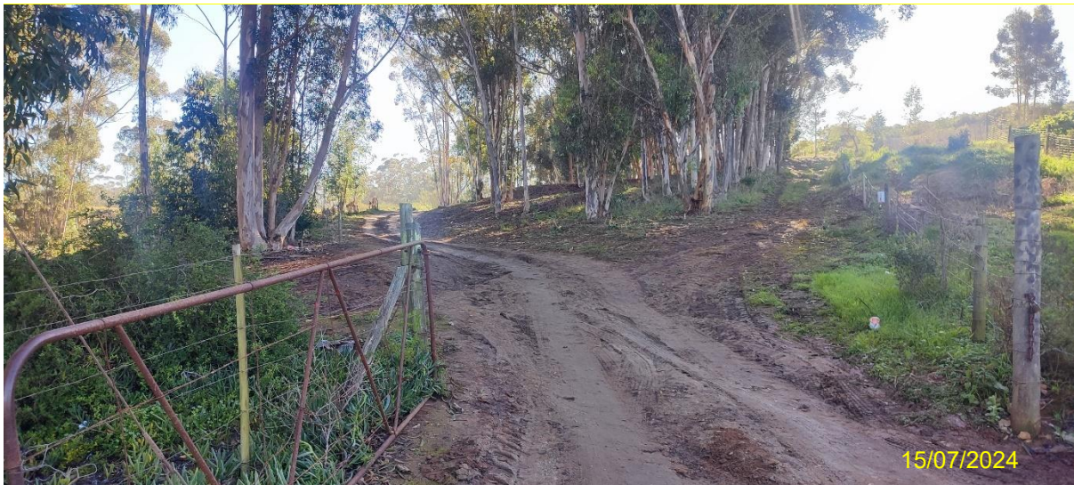
Photo 1: Existing access road off Muir Street to water treatment works site which will be upgraded/formalised to accommodate construction and maintenance vehicles. The eucalyptus trees to the right of the access road are to remain to mitigate visual impacts of proposed water treatment works on adjacent homeowners and to stabilise the gradient.
