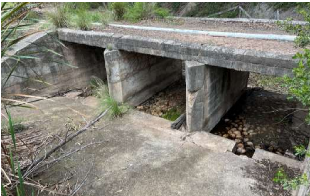
Figure 4-9: Looking downstream along spillway discharge channel
