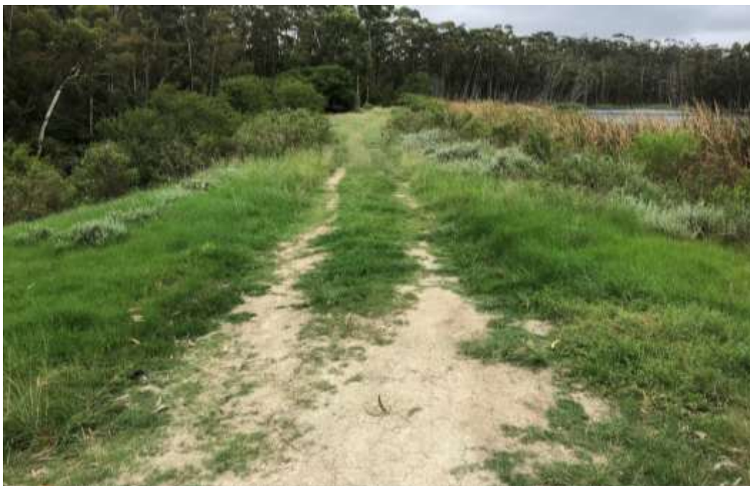
Figure 4-2: View of embankment crest from the left abutment
