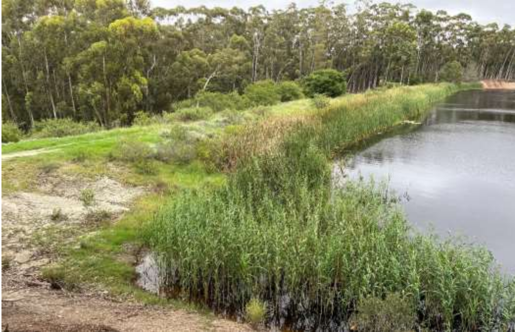
Figure 4-4: View of the upstream face from the left abutment
