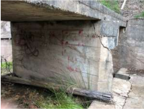
Figure 4-10: Damaged concrete channel walls
