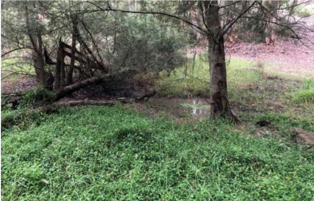
Figure 4-7: Audible stream and ponding at downstream toe
