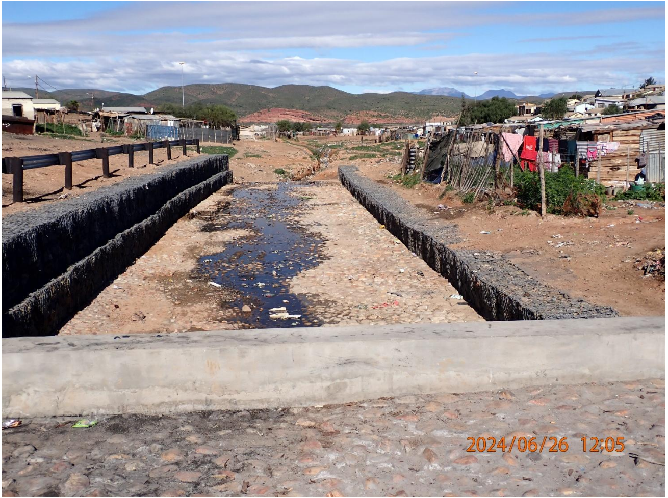
Photograph 13: Upstream view of drainage line to be formalize.
