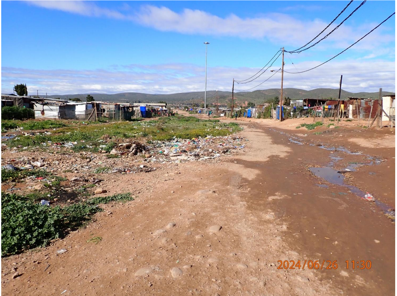
Photograph 8: Road that followed the route of the original stream. Water flow in and next to road.
