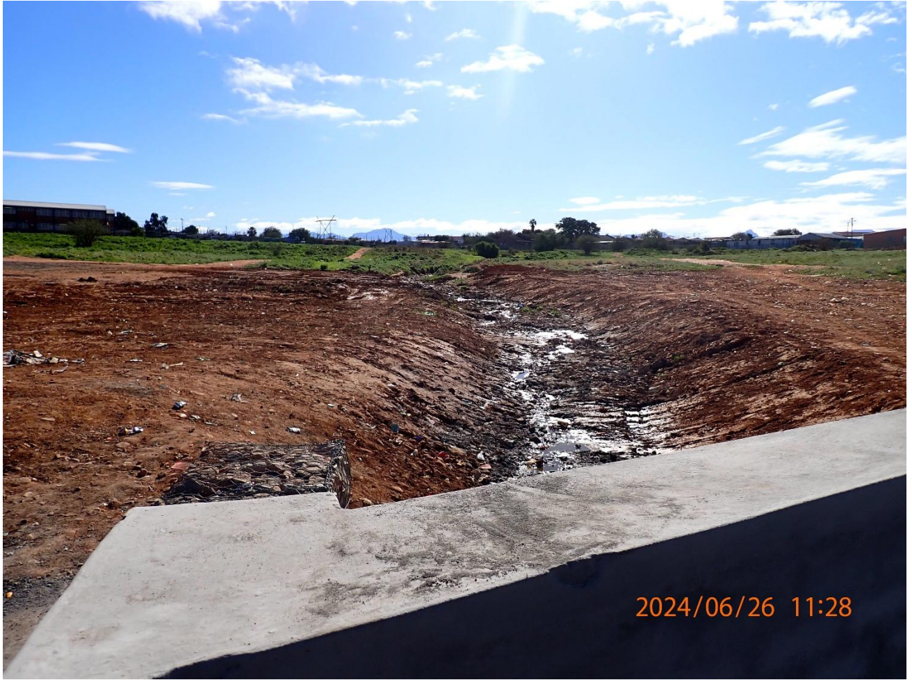
Photograph 5: Upstream view of formalized stream.
