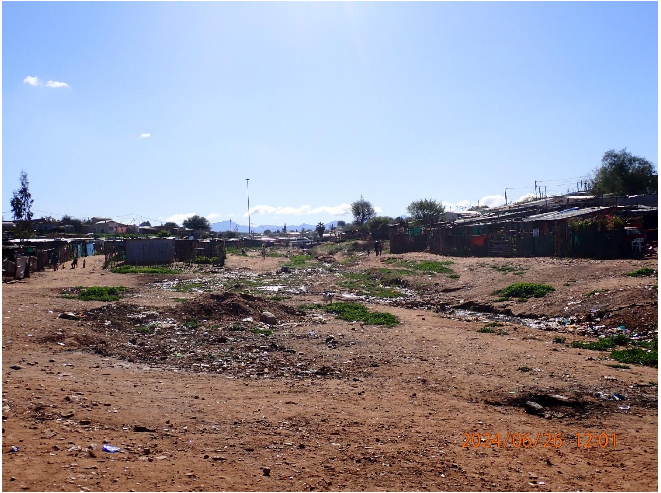
Photograph 15: Ecological condition of original stream that will be formalized.
