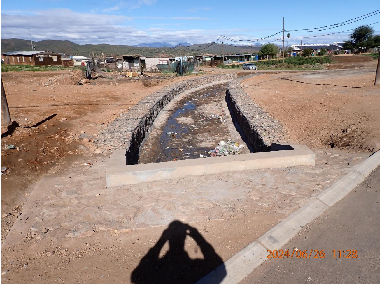
Photograph 6: Upstream view of formalized stream.
