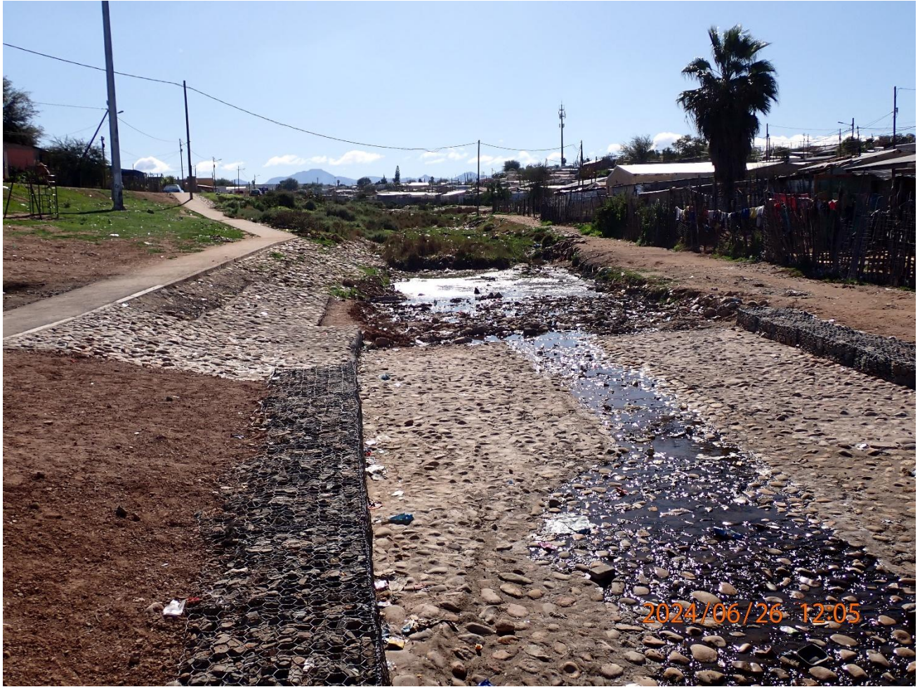
Photograph 14: Upstream view of drainage line.
