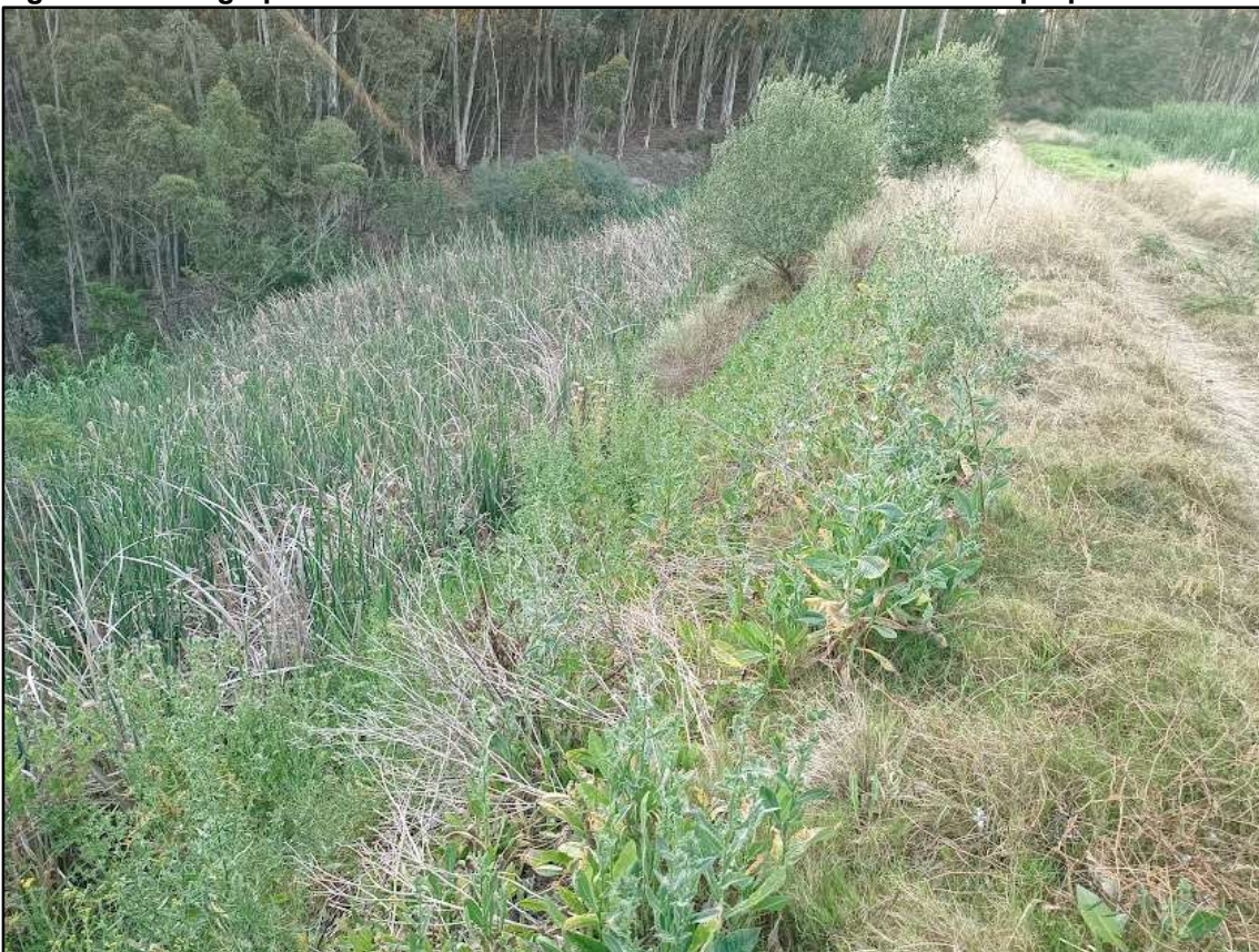
Figure 7: The dam wall of the reservoir showing evidence of an “incidental” or man-made wetland (due to the presence of Typha capensis ) due to seepage from the dam wall.
