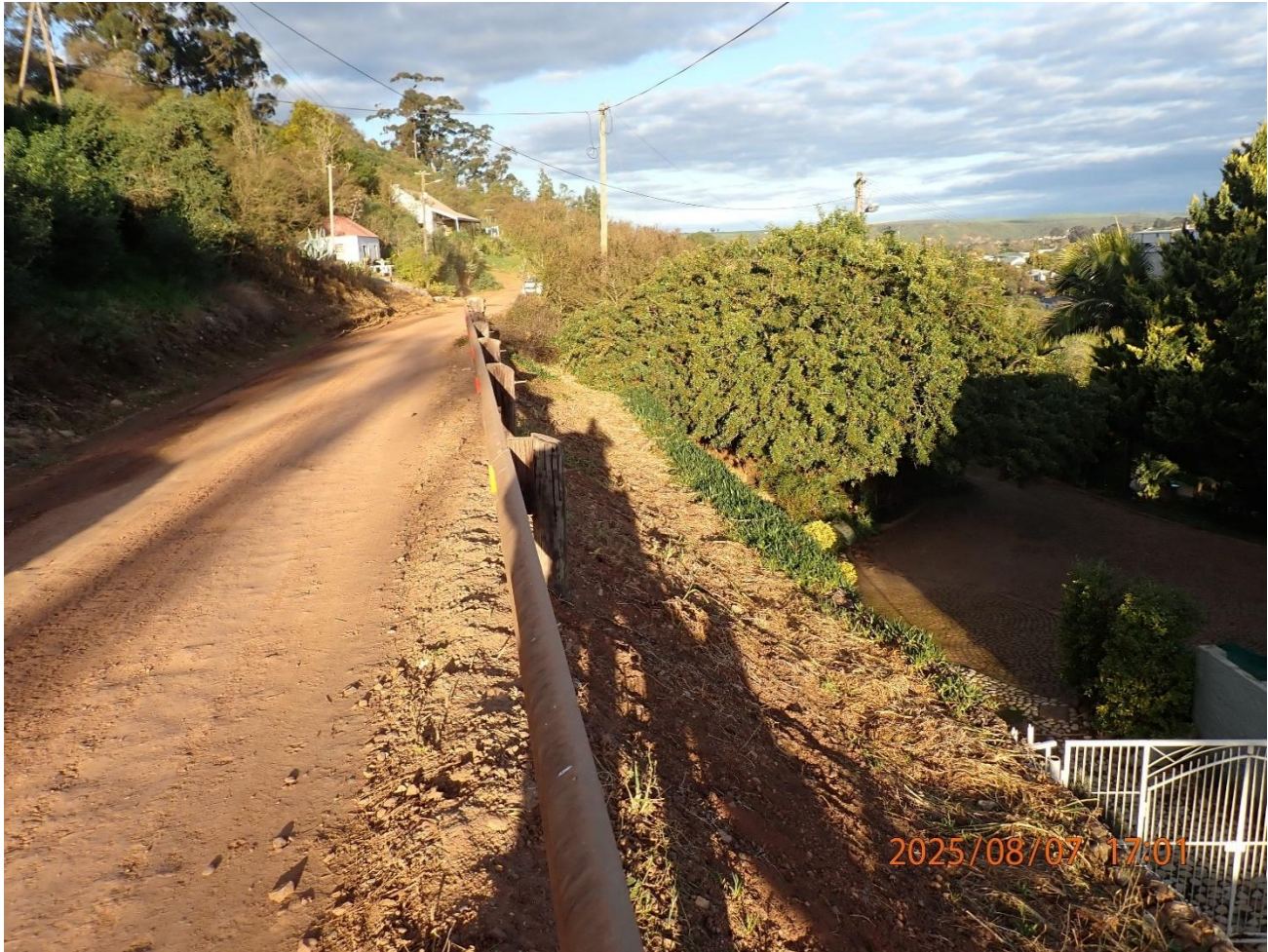
Photograph 10: Proposed pipeline connection route.
