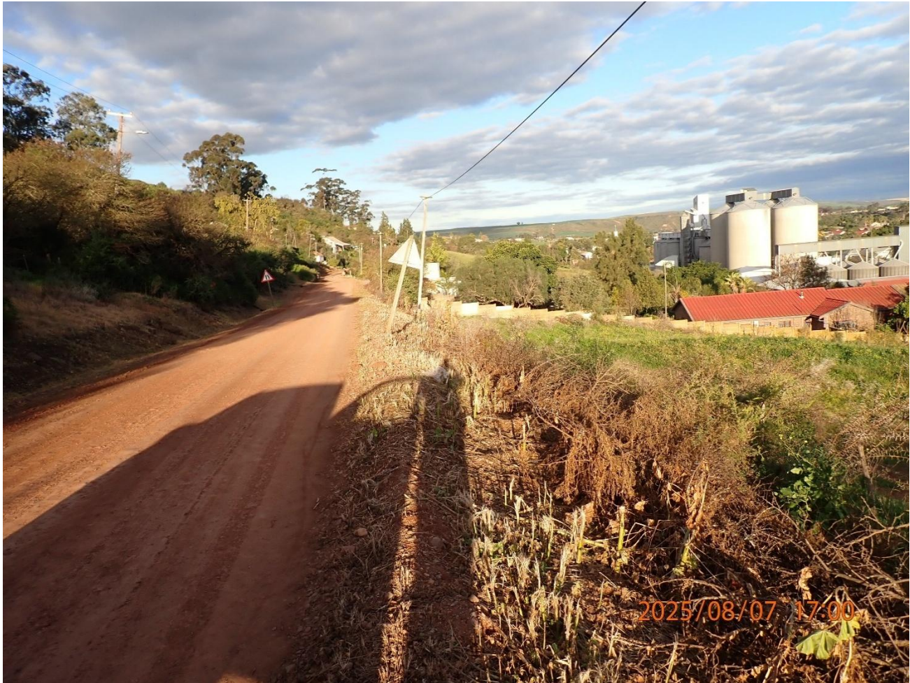
Photograph 11: Proposed pipeline connection route.
