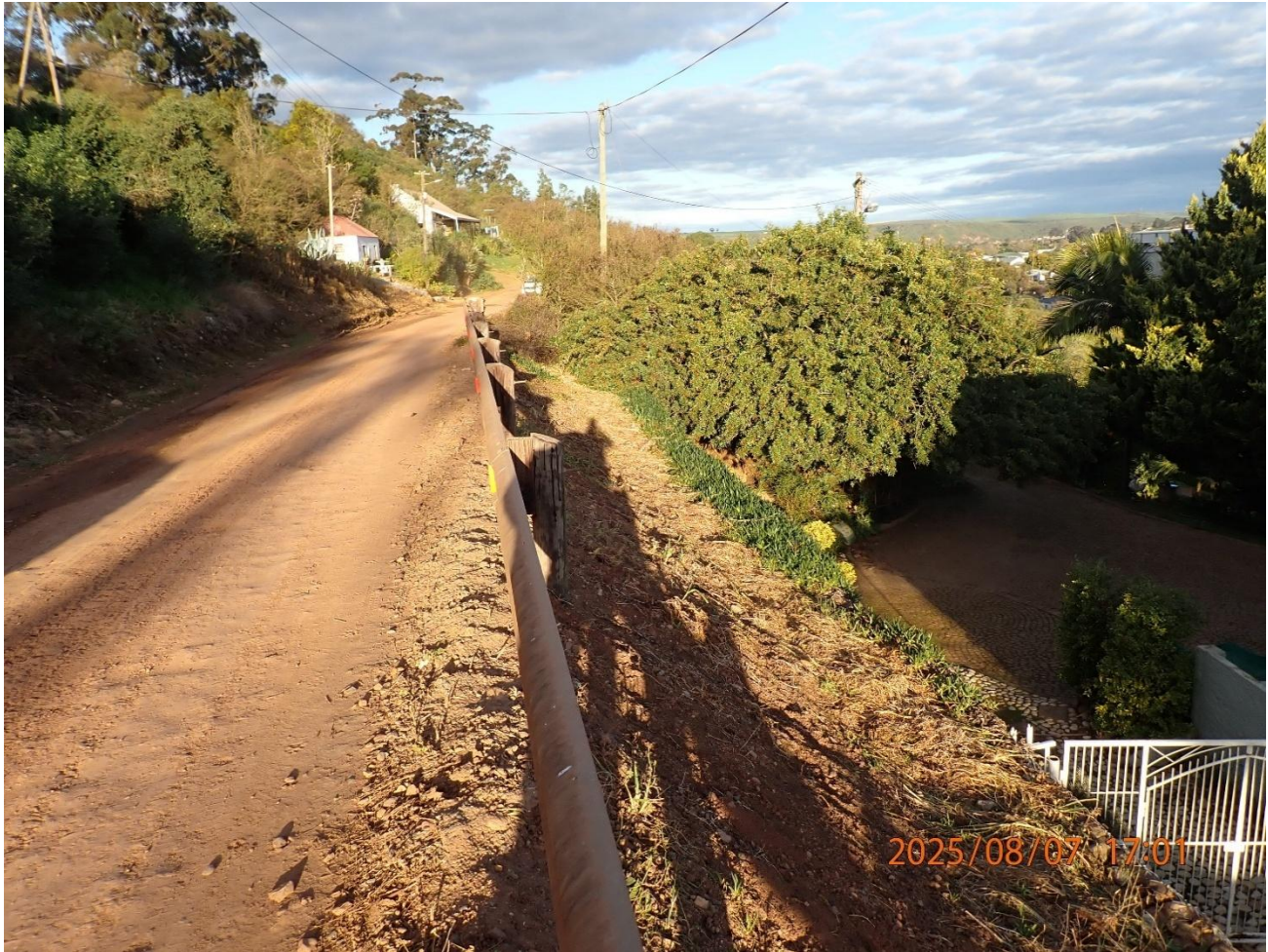
Photograph 6: Proposed pipeline connection route.
