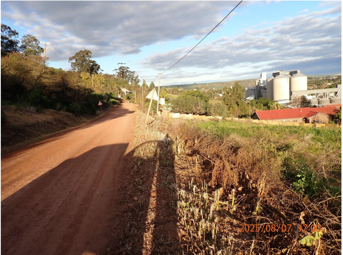
Photograph 7: Proposed pipeline connection route.
