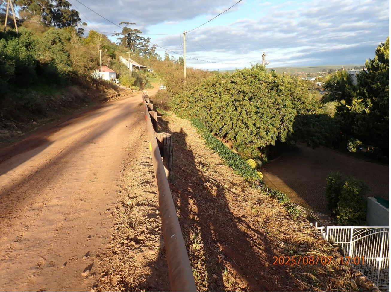
Photograph 6: Proposed pipeline connection route.
