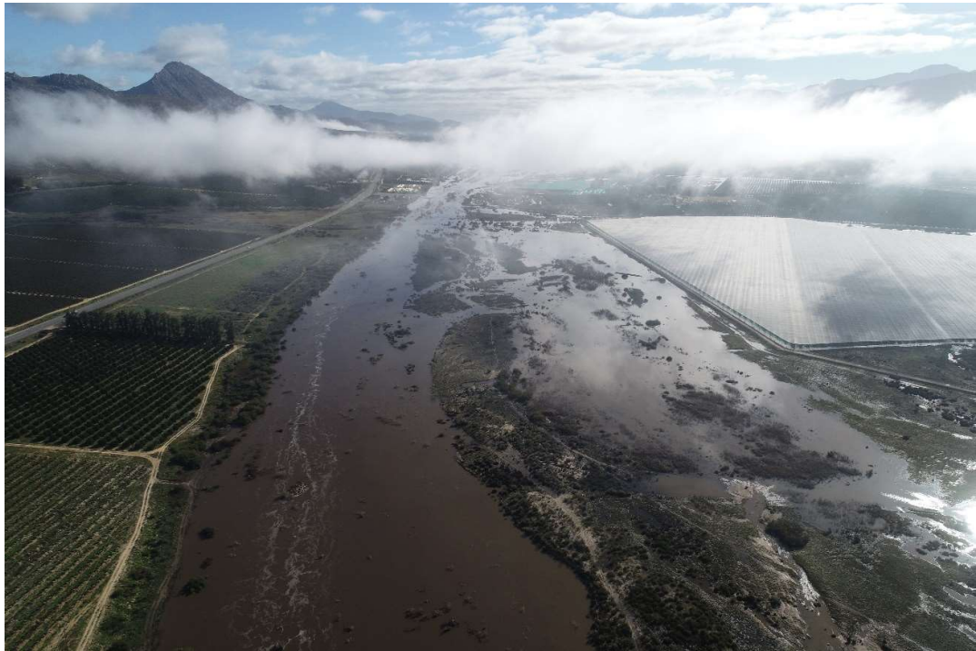
FIGURE 2: FLOODING OF OLIFANTS RIVER IN JUNE 2023
