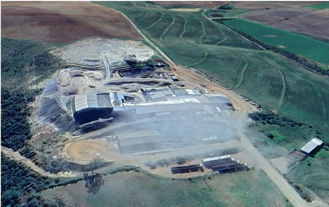
Figure 1 Applicants plant in Heidelberg showing dust above facility
