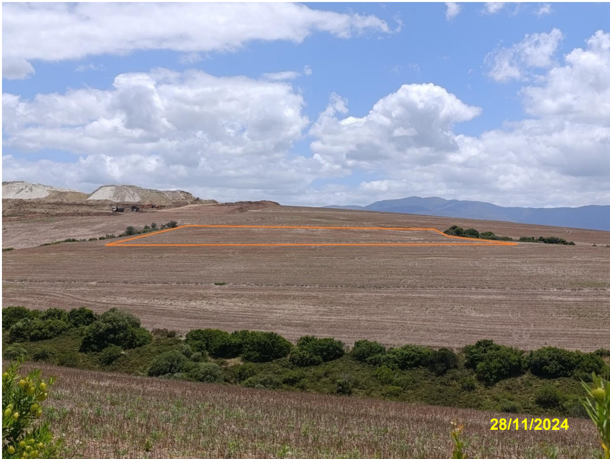
Site Photo 1: Phase 8 additional quarry proposed within approved mining right area on transformed cultivated land of Farm Rest van Uitspanskraal RE/585.
