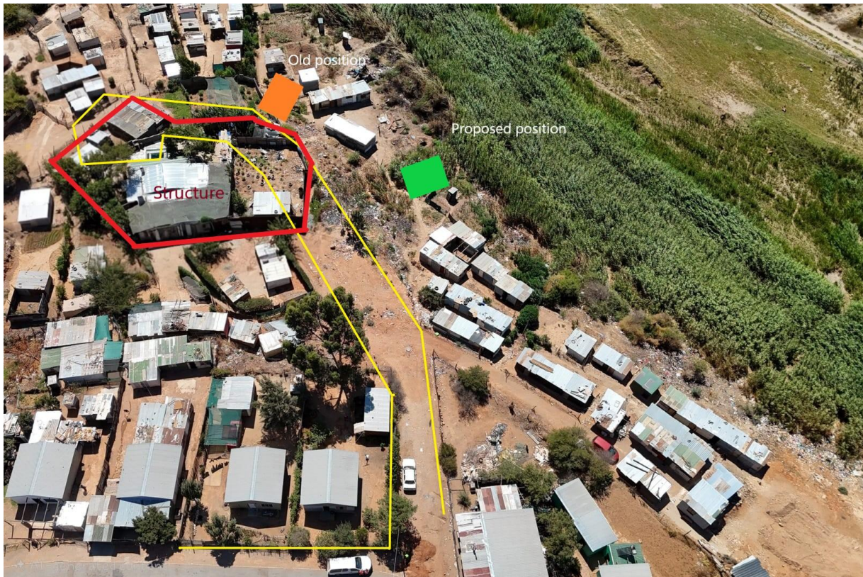
Photo 1: Aerial photo of informal structure which the owner is refusing to remove and old position of proposed stormwater outlet (orange square) and new proposed position of stormwater outlet (green square) at Mandela Square informal settlement.
