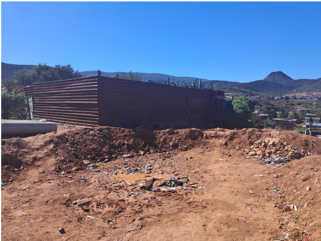
Photo 2: Informal structure in the way of original stormwater outlet location.
