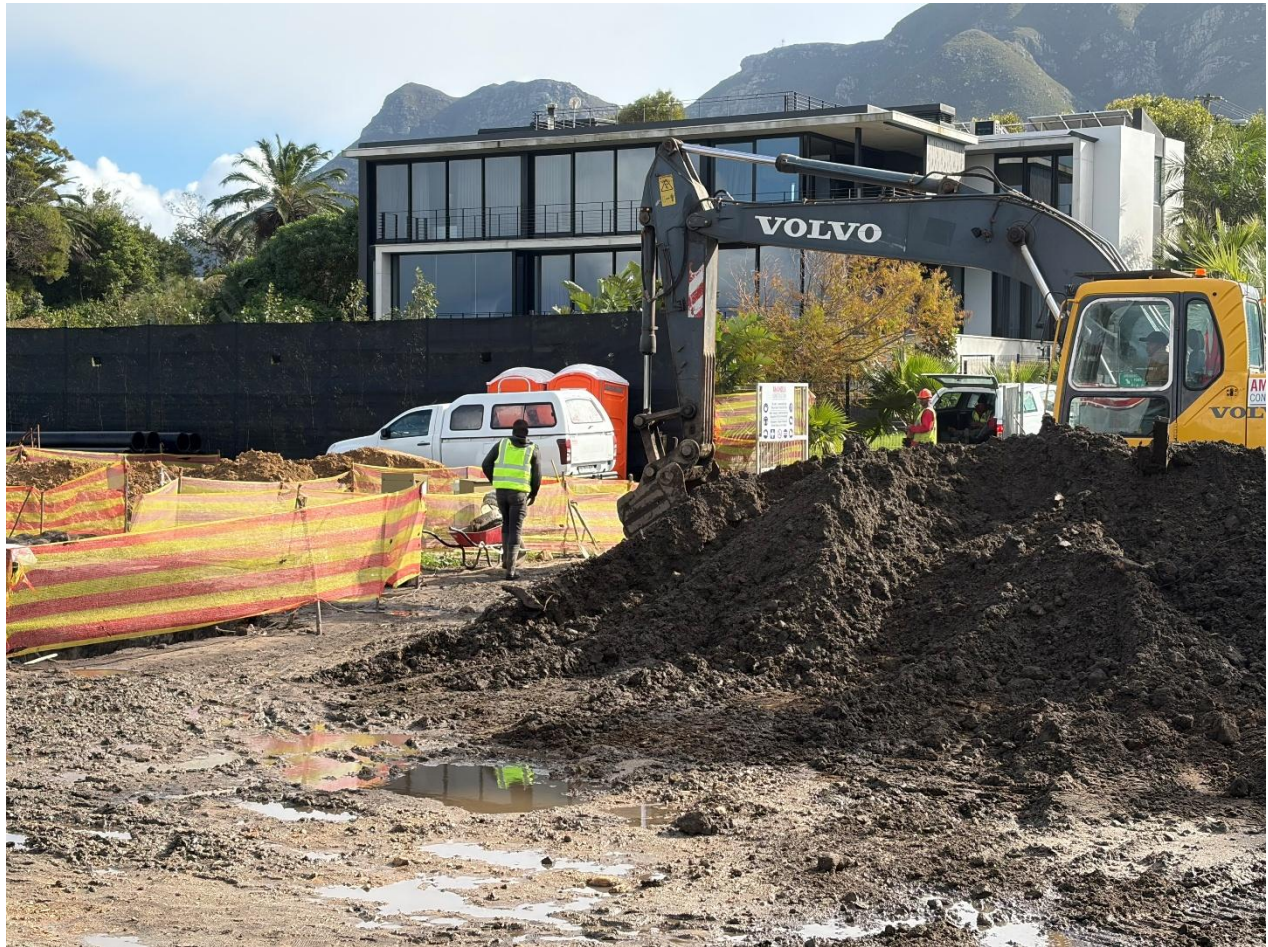
Photograph 5: Construction activities and toilet facilities.
