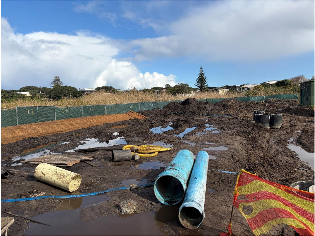
Photograph 6: Construction activities and site demarcation with berm.
