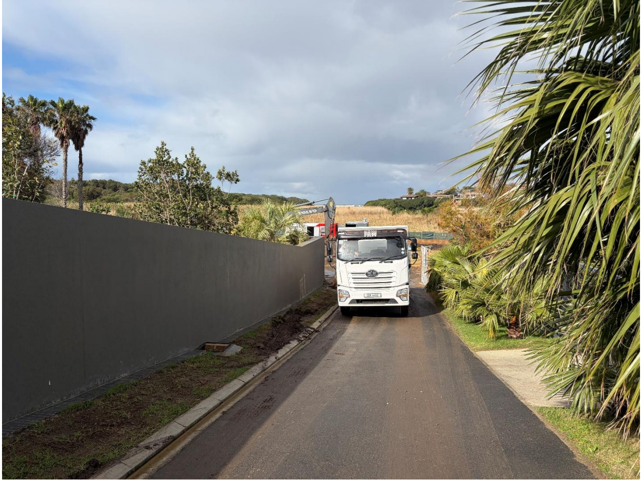
Photograph 1: Access to construction site.
