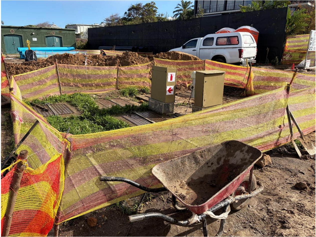
Photograph 10: Construction activities and demarcation of existing infrastructure.
