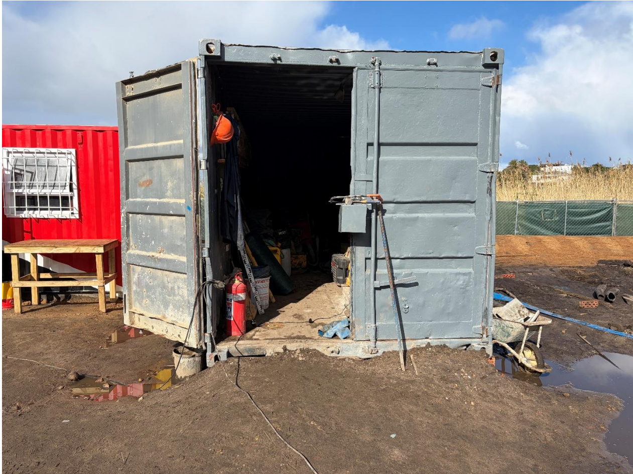
Photograph 11: Container on site to store construction equipment.
