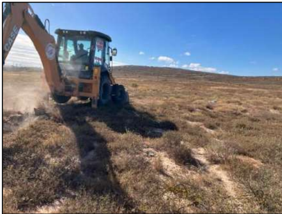
Plates 9 & 10: Test pits mostly refused at relatively shallow depths on the very dense dorbank, in some areas beneath the site
