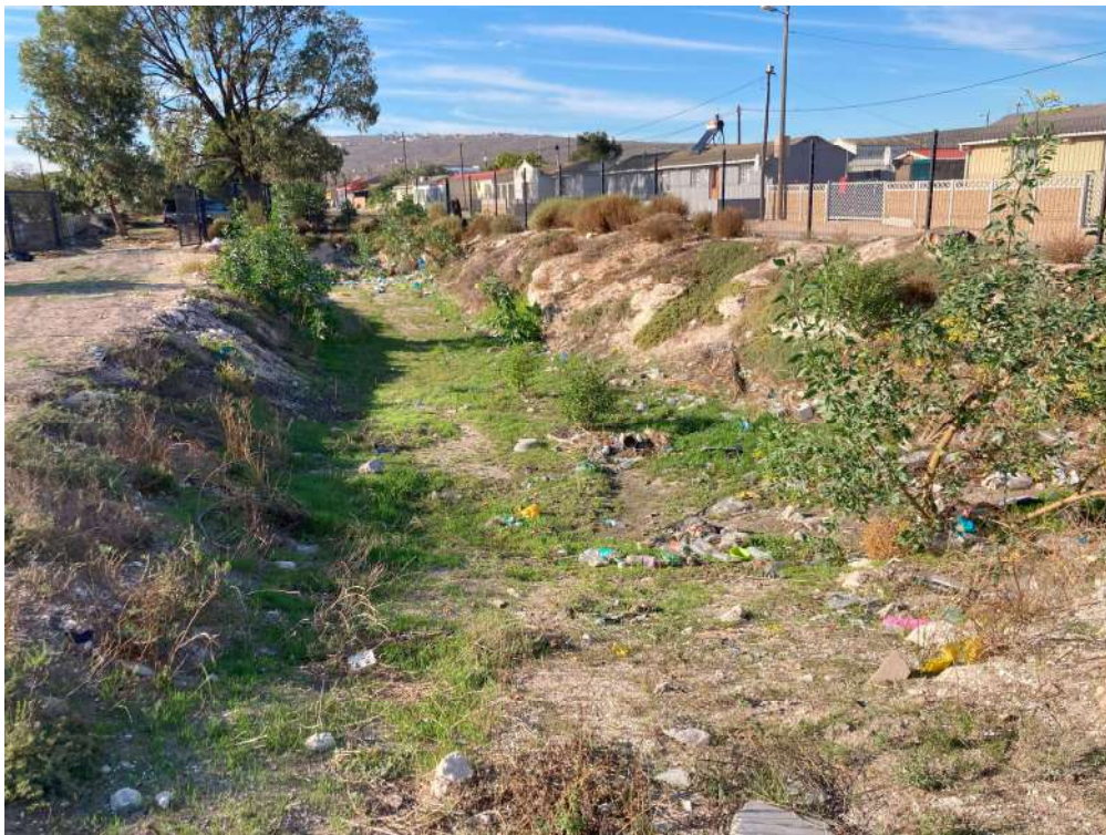
Figure 2: Existing attenuation facility at the intersection of Minor Road 7664 and Main Road 00533
