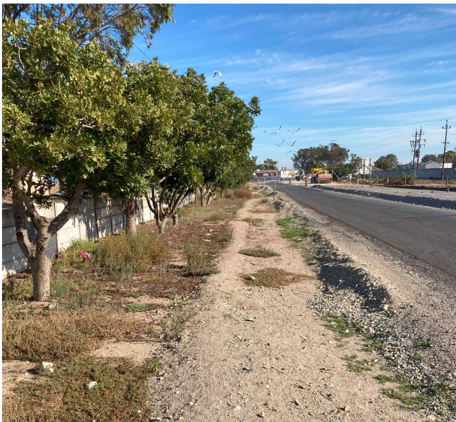
Figure 3: Main Road 00533 adjacent to the existing attenuation facility
