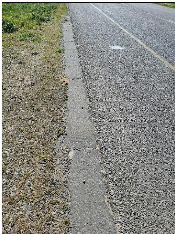
Pic 5 – View of concrete edge beam on Farm access/Haul Road access on R304
